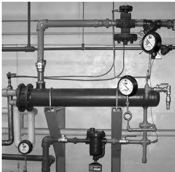
Feedback instantaneous systems may suffer from lag time, tube bundle corrosion and problems with thermostatic element deterioration.
